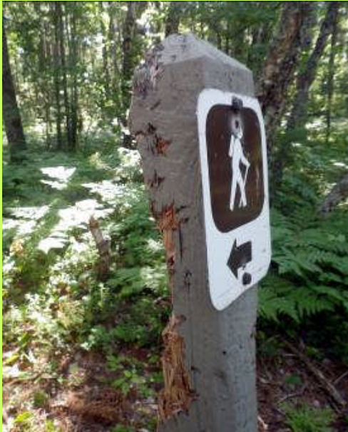
Bear Damage—Stockton Island
